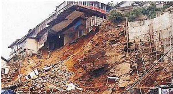
Fig 2.6.1 Landslide in hilly terrain of India
